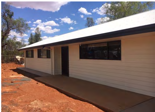
Rebuild in Cobar Project Managed by MLAHMC
