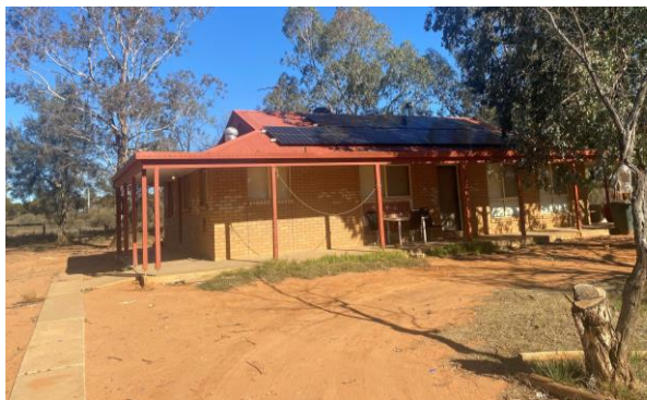
Solar panels installed to 48 Dareton LALC properties
